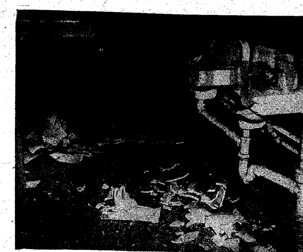
SMASHED WASH BASINS ACT AS MUTE EVIDENCE OF VANDALS' TRICKS These Costly Toilet Fixtures, Located in Unoccupied Harmony Church, Are Beyond Use Now
