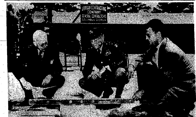
CUSTER ROAD CONSTRUCTION LAUNCHED WITH CORNERSTONE CEREMONY Left To Right, R. E. Matheson, Maj. Gen. W. A. Burreas, G. Gunby Jordan Square And Level Corner Of First Building In Multi-Million Dollar Project.
